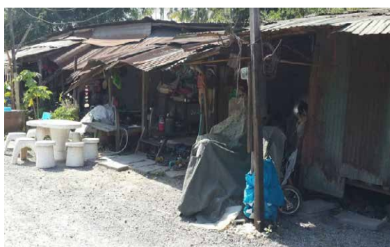
Workers' accommodation before renovation
