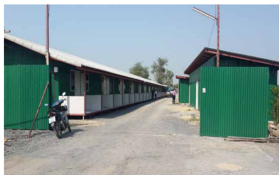
Workers' accommodation after renovation
