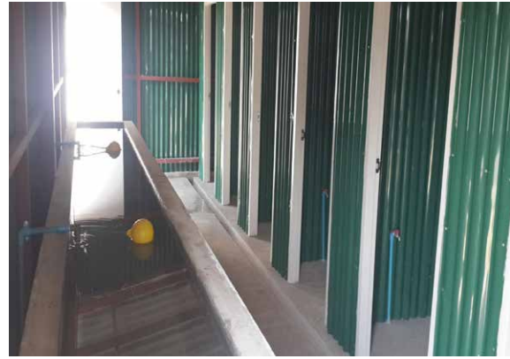
Toilets after renovation
